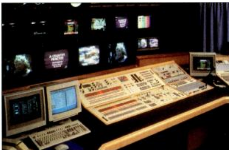
Pro-Bel's top-of-the-line Compass automation system
